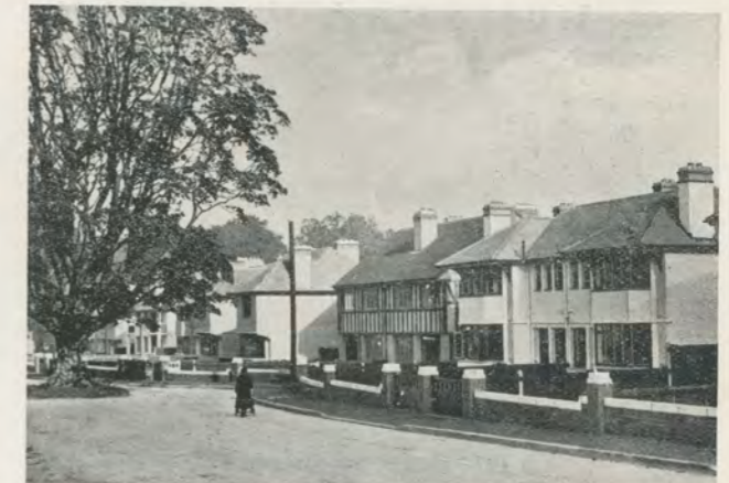
A completed road. Note how the beautiful Park timber is preserved.
