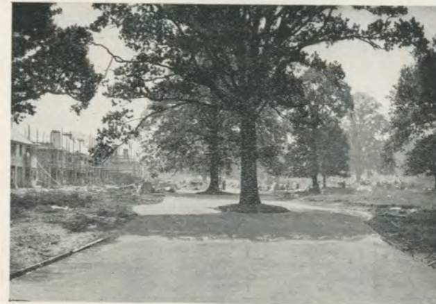
The opening of the Estate with houses in progress and roads in course of formation.
